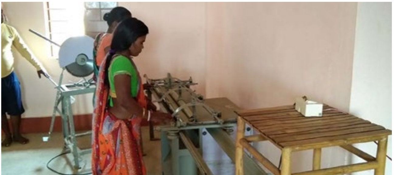
Women artisan working after installation of solar power unit
